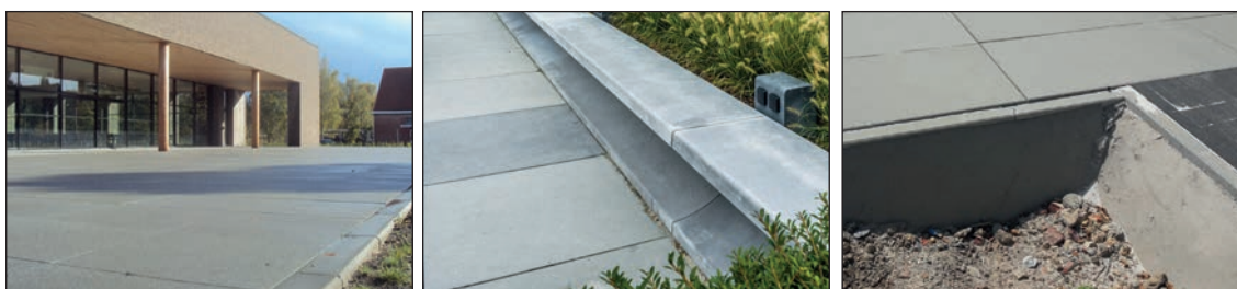
Figure 9.1 – Contrebutage correct:
